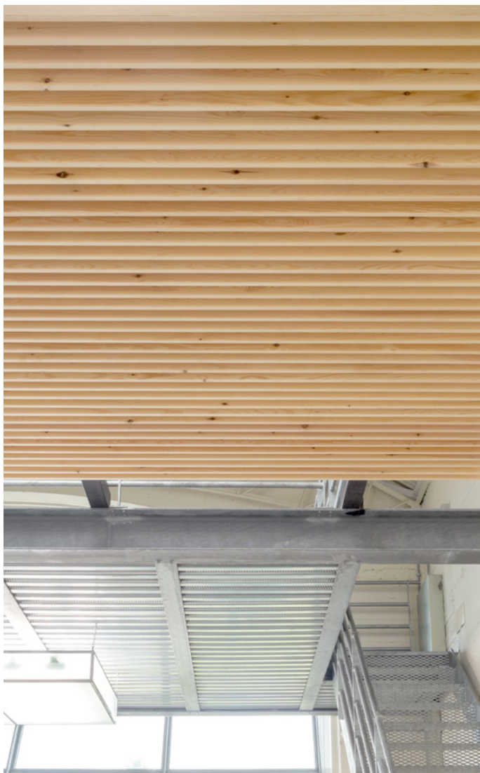
Top left and below details of a natural spruce false ceiling; above details with a lacquered finish.
