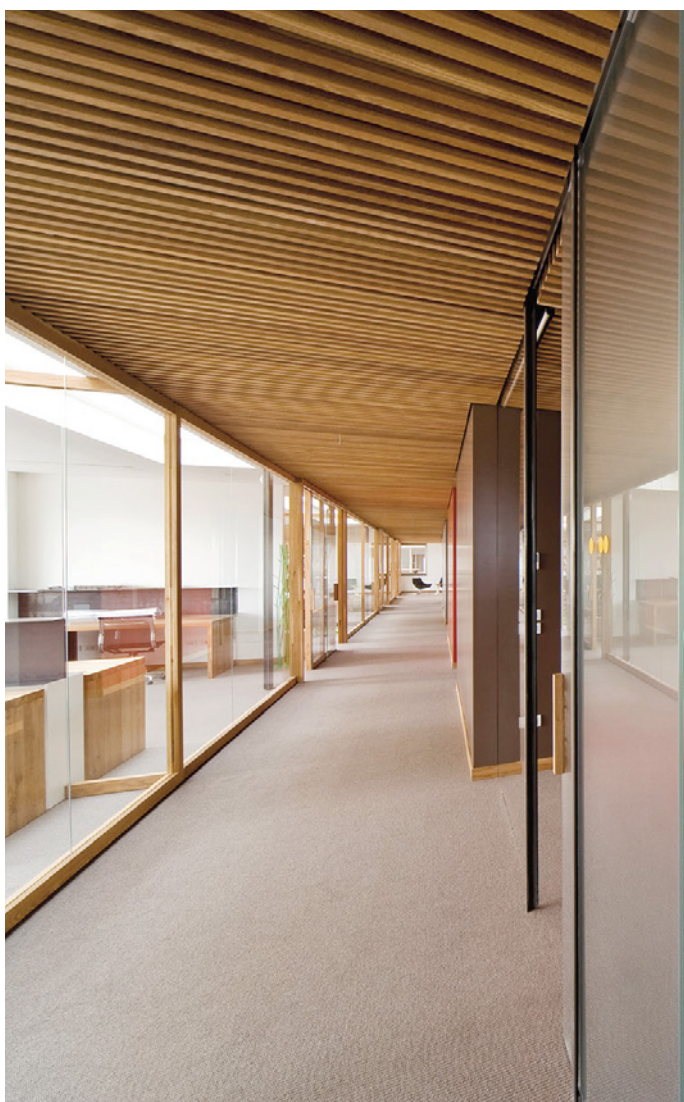
Details of oak slats with an oil finish.
