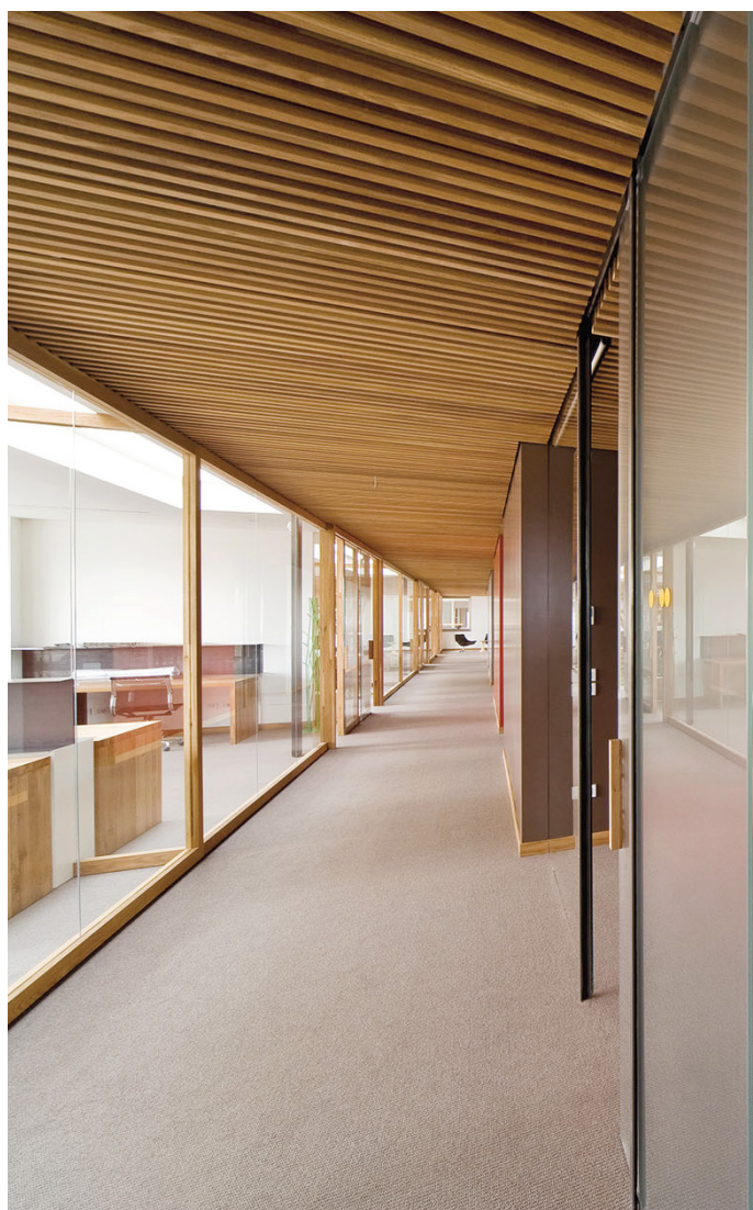
Details of oak slats with an oil finish.
